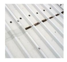
the metal roofs of many of its premises. The problem was cut edge corrosion. It is caused by a combination of poor installation techniques and on-site cutting plus attack from acid rain and pollutants, which are then retained as moisture in critical roof overlaps and gutter overhangs. This results in corrosion of the profiled steel roof sheets. If not treated quickly and effectively, the damage can often lead to the need for partial or complete roof replacement. Seamsil provides an
